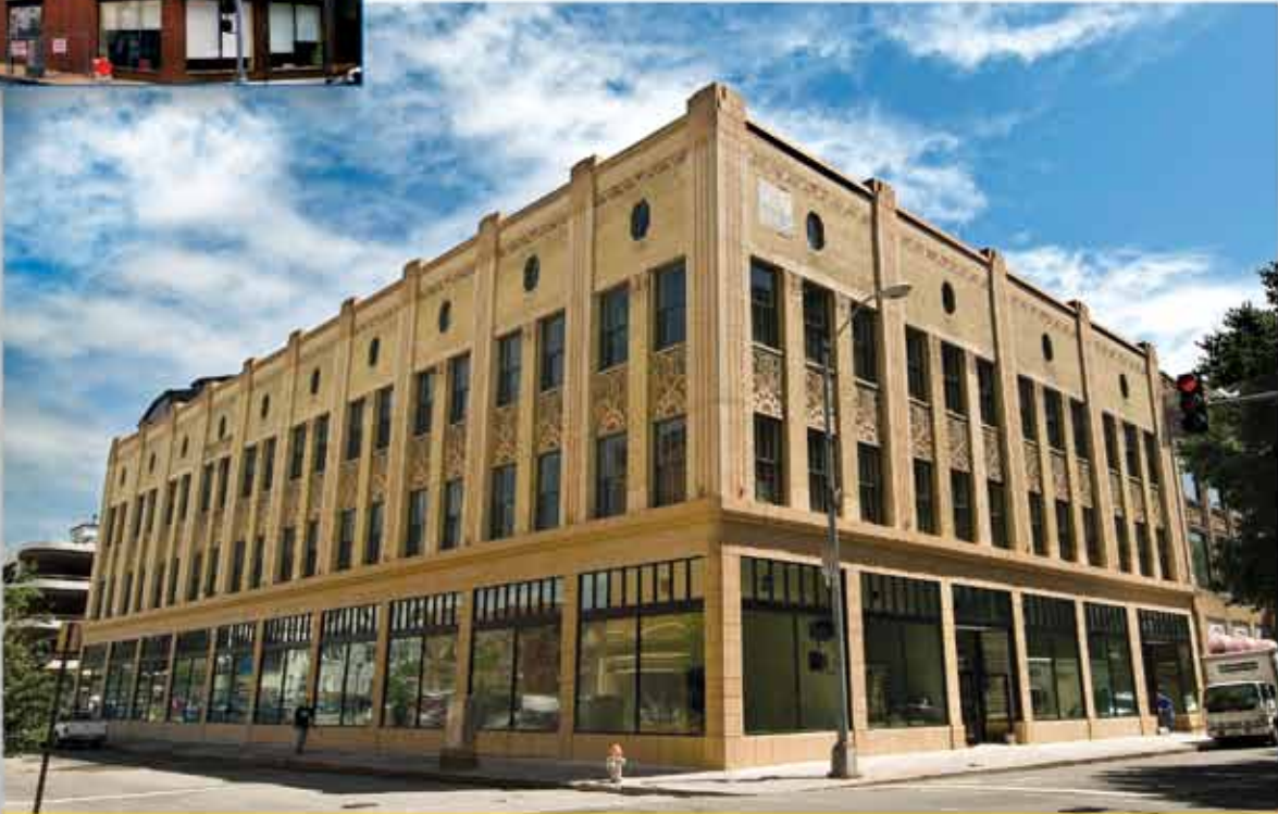
After - The Hancock Building in Roanoke, Virginia
