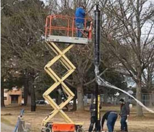
IN FEBRUARY THE CITY OF HAMPTON completed the installation of fifteen solar-powered smart poles as part of its “Digital City Transformation” initiative. The poles will provide Wi-Fi access, charging ports, and lighting for enhanced security to the Y. H. Thomas Neighborhood Park. The poles can store energy for up to eight days with no sunlight and are designed to light the area where someone is walking, both to save energy and to reduce light pollution.
