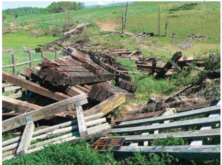
The 2011 tornado destroyed the 636-foot long trestle five miles south of Abingdon on April 28, 2011. With the help of VML Insurance Programs, a new 454-foot long trestle was built in its place with 34 steel-reinforced concrete footers, as well as two steel-reinforced concrete abutments as the foundation. The total cost of the claim for VMLIP was $2.2 million.
