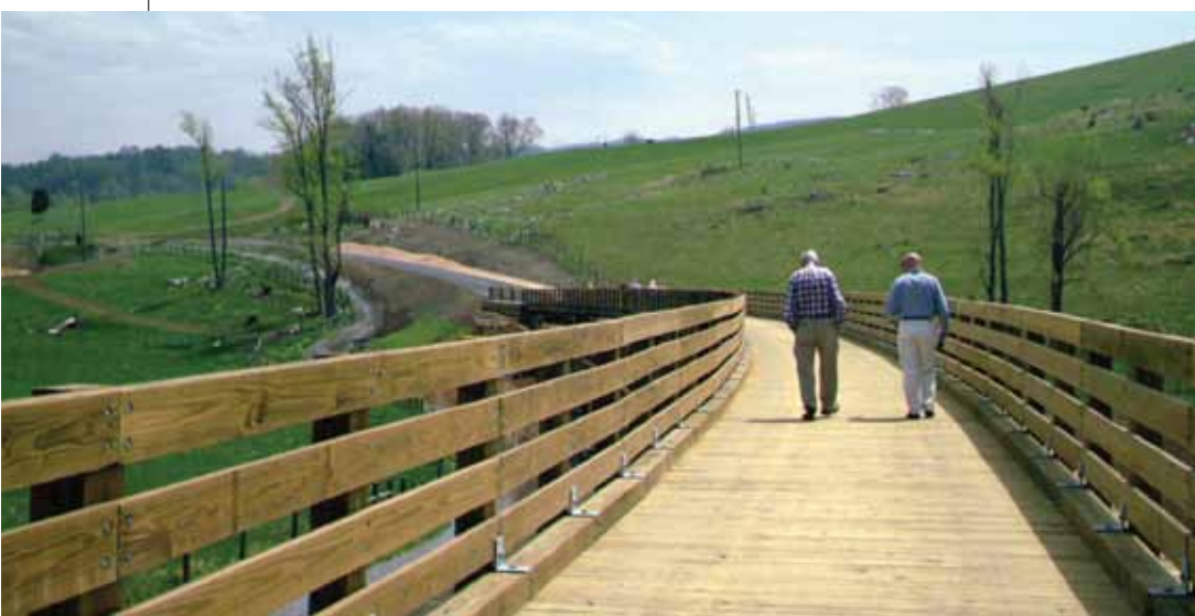
The 2011 tornado destroyed the 636-foot long trestle five miles south of Abingdon on April 28, 2011. With the help of VML Insurance Programs, a new 454-foot long trestle was built in its place with 34 steel-reinforced concrete footers, as well as two steel-reinforced concrete abutments as the foundation. The total cost of the claim for VMLIP was $2.2 million.
