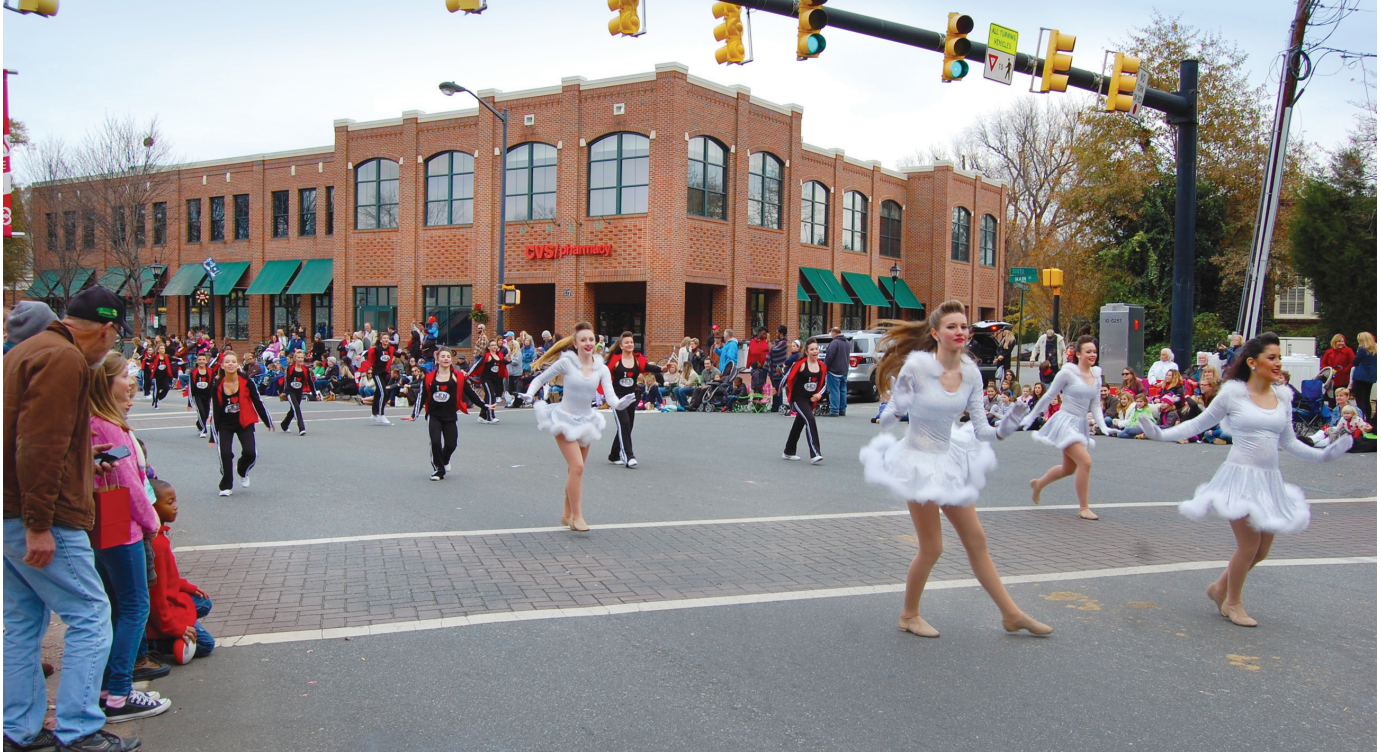
When CVS proposed building a new store in Davidson, North Carolina, the town insisted on a two-story brick building, pulled to the corner with parking in the rear. The result is a building that fits into the fabric of the community.
