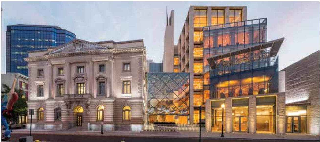
The Mid-Atlantic Chapter of the American Public Works Association honored Norfolk's Department of Public Works for its role in construction of the new Slover Library.
