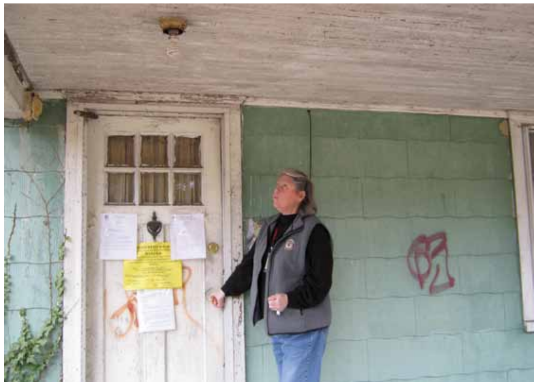
Chesterfield County Property Maintenance Inspector Bonnie Johnson made numerous calls to plumbing companies to find volunteers to repair Kenny Oney's condemned home.
