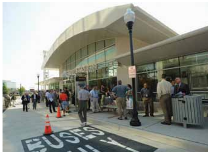
The Shirlington bus station serves more than 2,000 daily commuters in the urban village of Shirlington, proof positive that transit-oriented development can be successful without Metrorail. The station also houses a Commuter Store.
