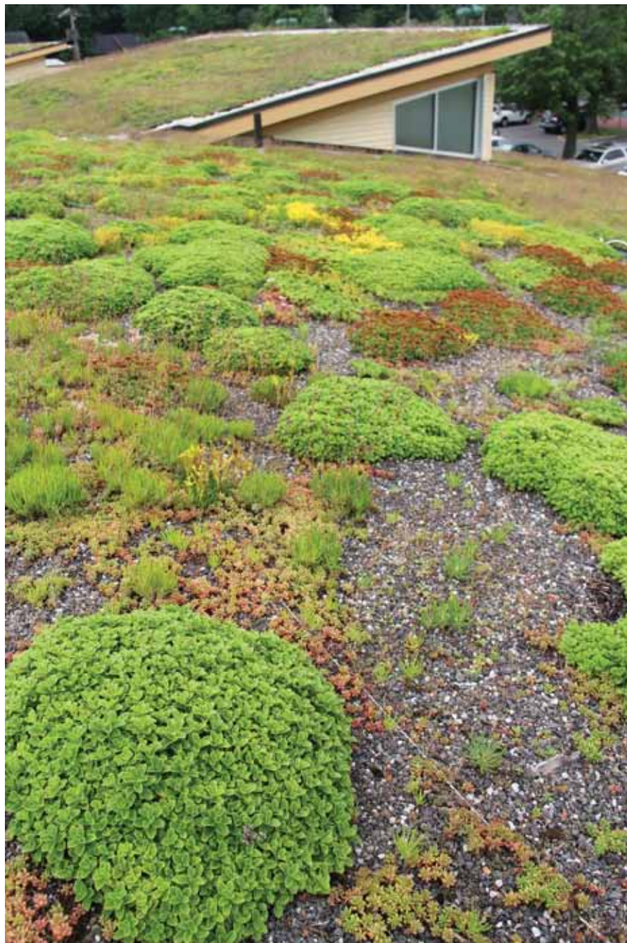
The green roof on the Walter Reed Community Center is one example of how Arlington's Initiative to Rethink Energy (AIRE) is helping to reduce emissions and lower costs.
