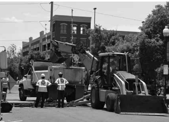
Utility relocation along Main Street is underway.
