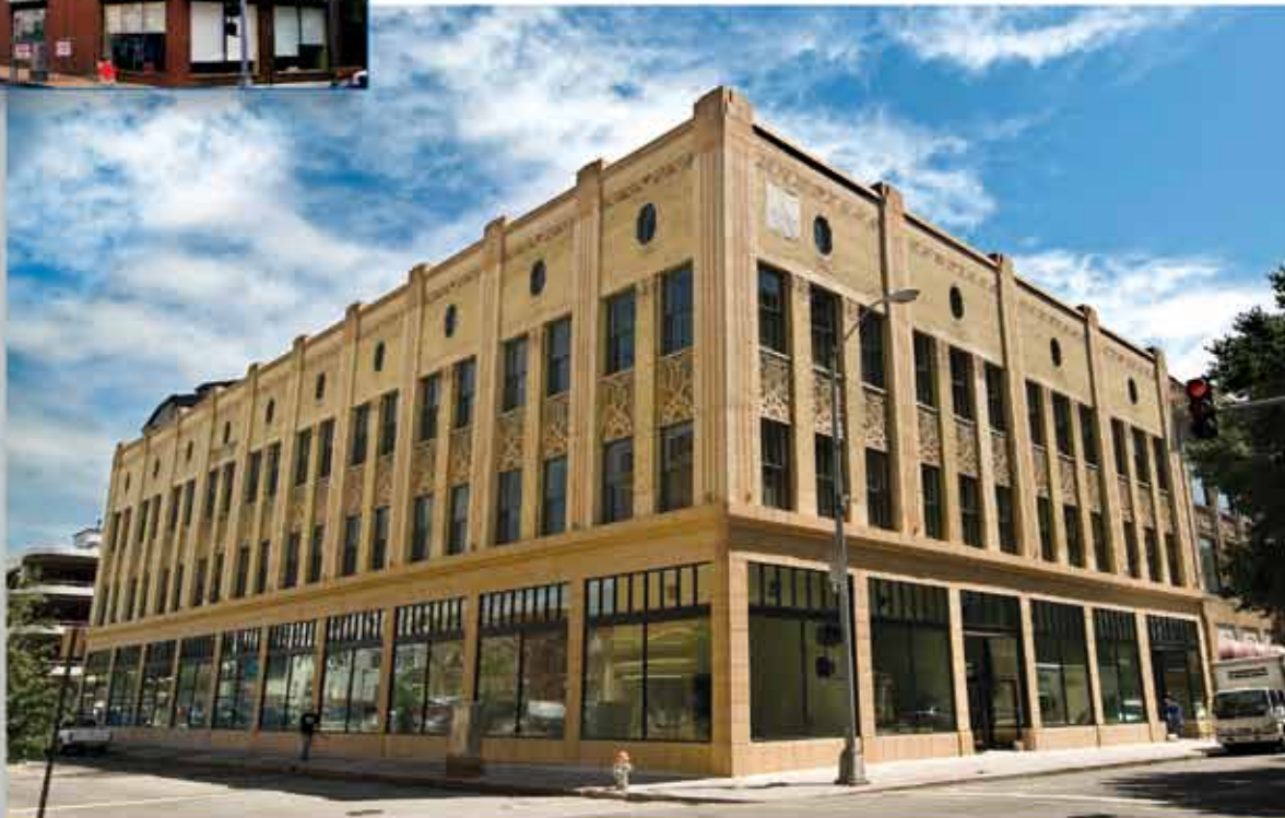
After - The Hancock Building in Roanoke, Virginia
