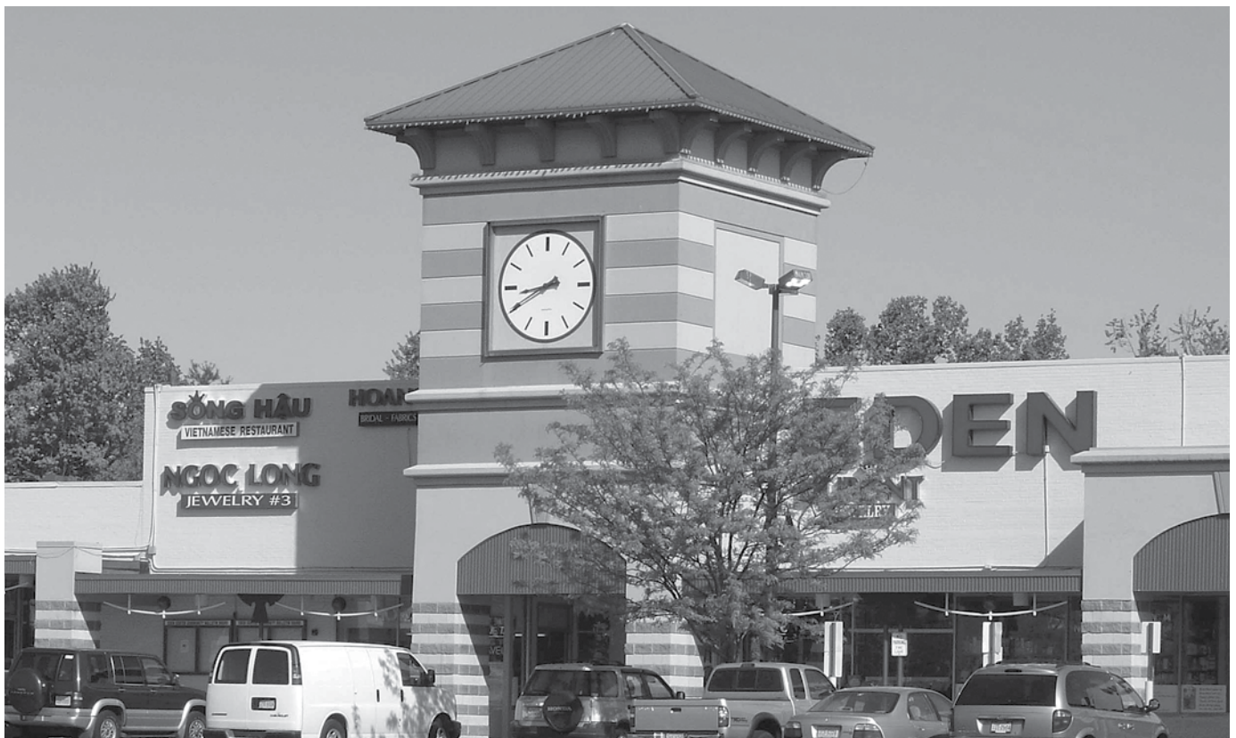
Inspection of the sprawling Eden Center Mall by the task force resulted in an assortment of health and safety violations that were discovered with a minimum of disruption to tenants.
