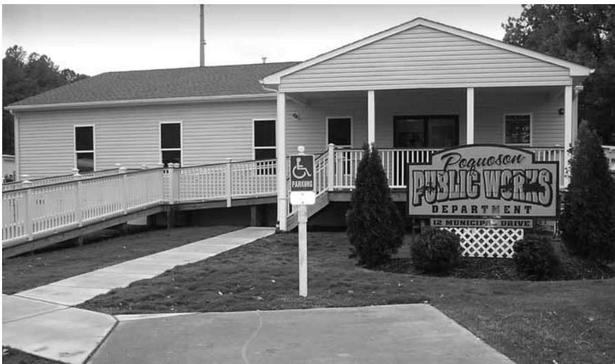
Instead of replacing the public works facility with another trailer, Poquoson built a permanent structure using city money and the more than $167,000 it received from VML Insurance Programs to replace the ruined trailer.
