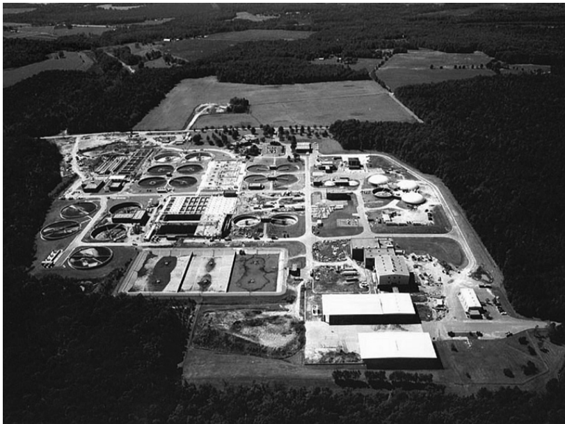
Henrico County is spending $86 million to significantly expand and upgrade the treatment capabilities of its Water Reclamation Facility.
